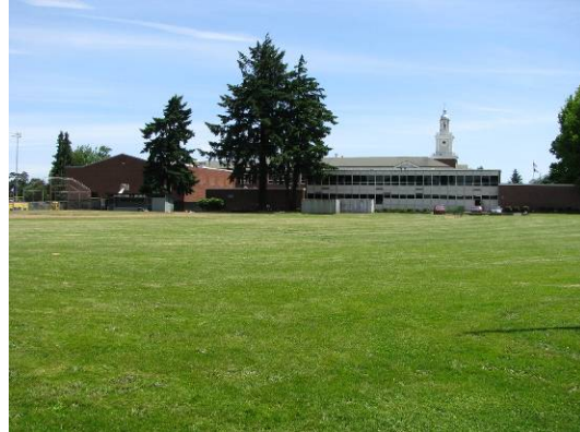
View from playing fields of west side of campus toward music and library addition (124E) and gymnasium addition (124D).
