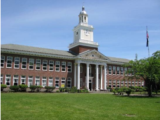
South elevation, main entrance (124A).
