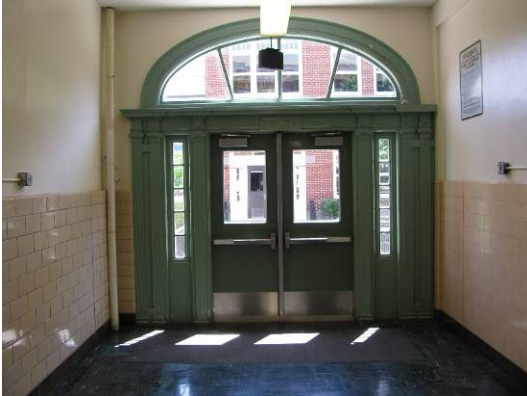
Typical ancillary exit from main building (124A).
