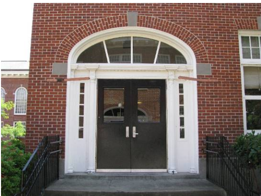
View of typical ancillary entrance, west elevation of main building (124A), looking toward auditorium (124C).
