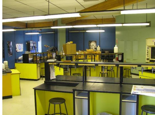
Classroom alterations on second floor of main building (124A).
