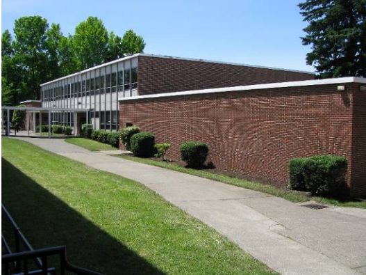
View of music and library addition (124E).
