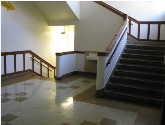
Stairway located near auditorium (124C).
